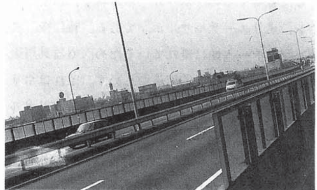
Photo14.5-4 Noise-barrier board on expressway (PC)
