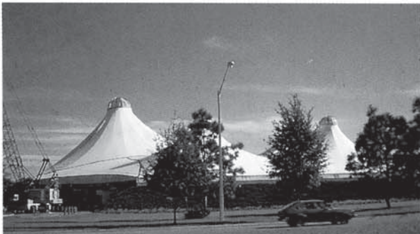
Photo14.5-3 Suspension-membrane structure (FR)
