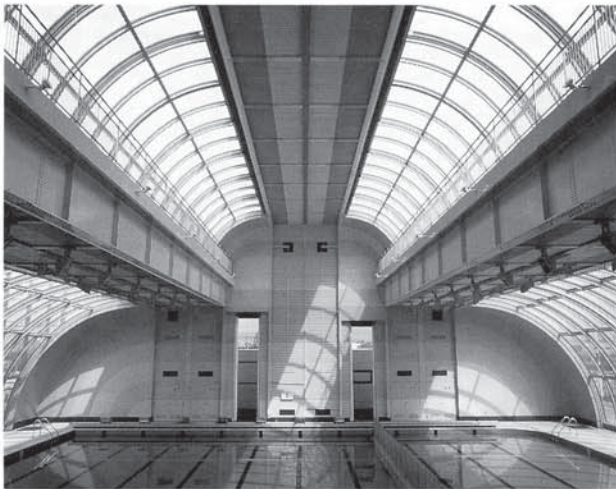
Photo14.5-6B Roof of indoor swimming pool (PC)
