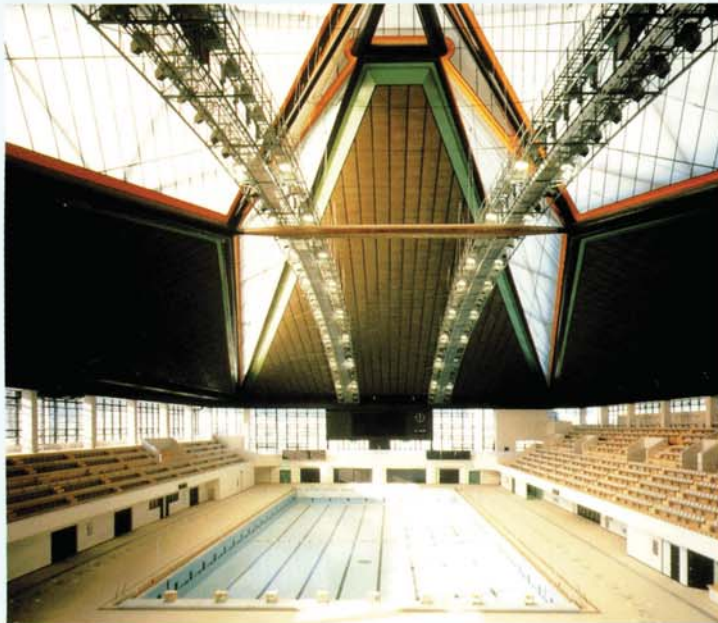
Indoor swimming pool roof (PC)
