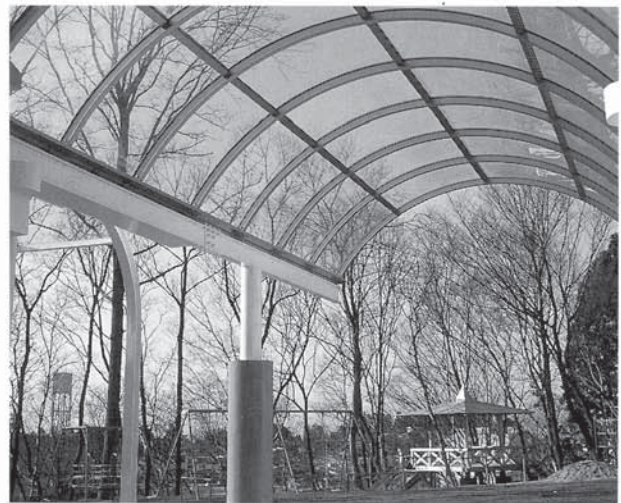
Photo14.5-5 Arcade parking place (PC)
